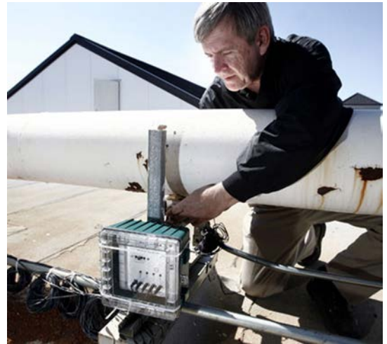
Pest control operator installing the Ultrason X, an ultrasonic bird control device.
